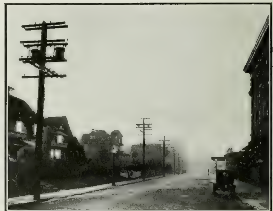
Disfiguring Poles at the Beach Avenue Entrance to Stanley Park.
